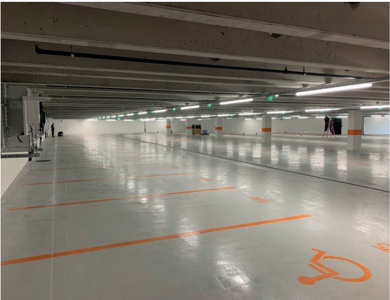
Image 4: Parking made easy: Highly pretensioned, prefabricated steel mats allow for floor spans of more than 17m.
