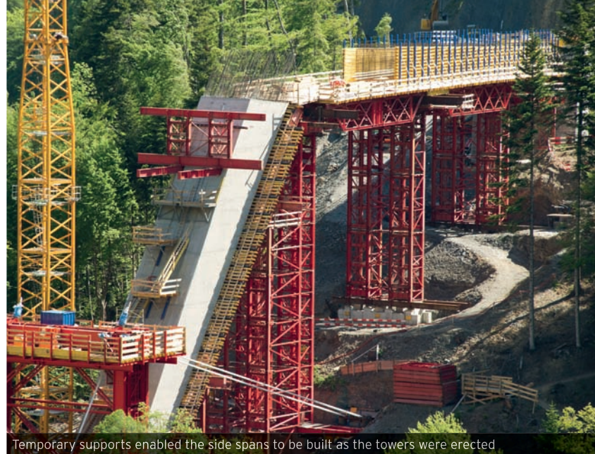
Temporary supports enabled the side spans to be built as the towers were erected
