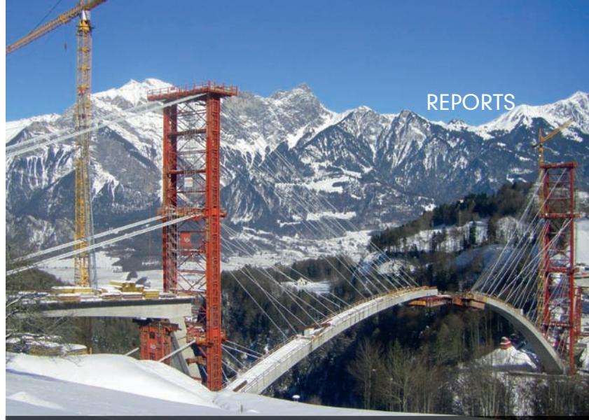
The temporary cables typically supported the arch every second segment
