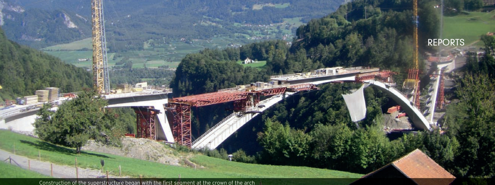
Construction of the superstructure began with the first segment at the crown of the arch
